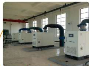
Sewage treatment plant in Hubei
